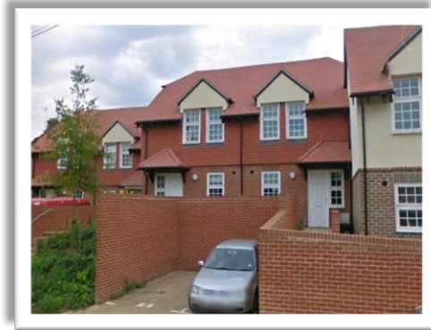
Windows manufactured and installed to a new housing estate in Guilford
