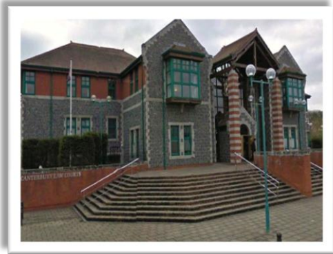
Window refurbishment to the Family Courts at Canterbury
