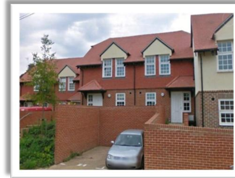
Windows – Guilford Housing Estate
