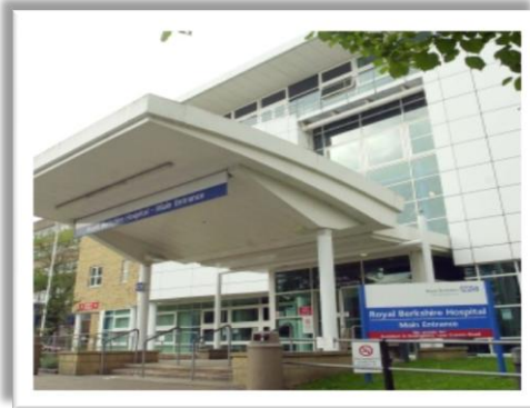
Royal Berkshire Hospital - Reading
