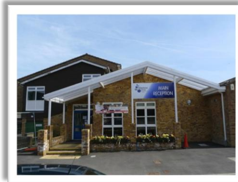
Reception Desk, Windows and Doors manufactured and installed to this school in Dartford
