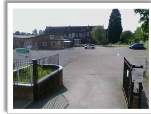
Suspended ceilings were installed here at a Adult Education Centre in Penge
