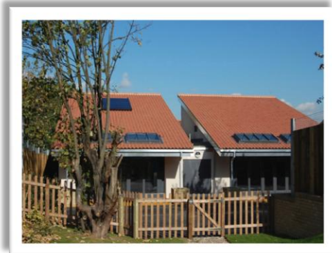
Windows and Furniture to this Children's Centre in Plumbstead
