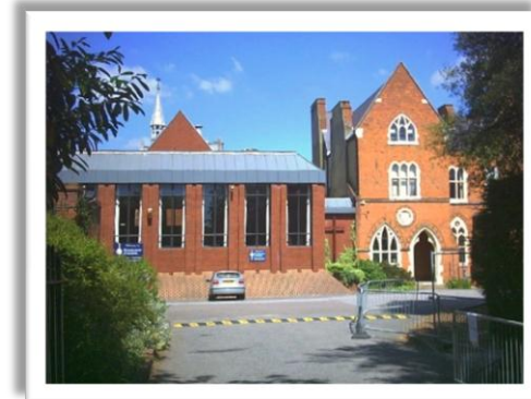
Windows and Doors manufactured and installed at this University in Wimbledon
