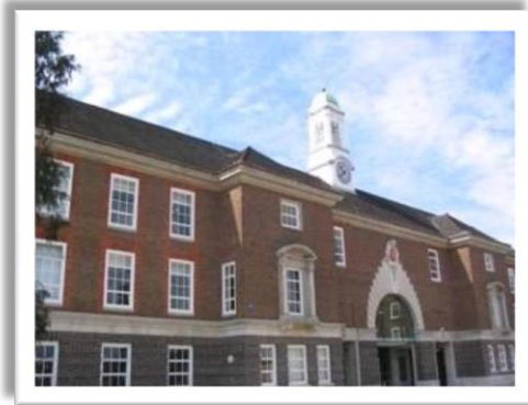
Furniture and Fire Doors manufactured and installed at this University in Hendon
