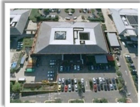
2 hour fire rated doors and frames manufactured and installed at Tesco
