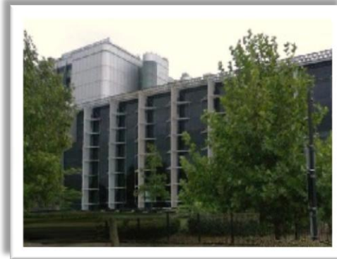
30FR-60FR-120FR Doors and frames manufactured and installed at Global Switch
