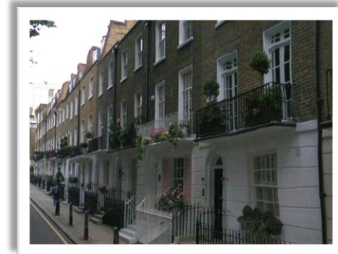
Fire doors and frames manufactured and installed to these homes in Knightsbridge
