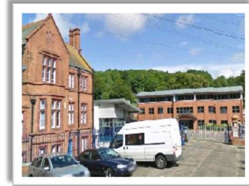
Joinery works at HMRC Dover
