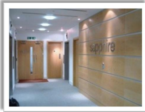
Panelled partitioning installed in offices at Lower Thames Street
