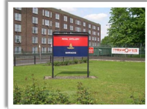
Focus E & Hygeine ceilings fitting at barracks in Woolwich
