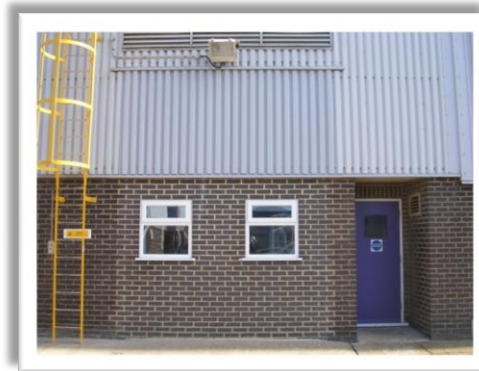
Matched brickwork extension at Kent Power Station
